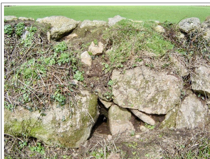
Typical rabbit entry in an old, poorly built hedge, as found on many 19th century miners' smallholdings. Easily blocked by knocking in a stone.
