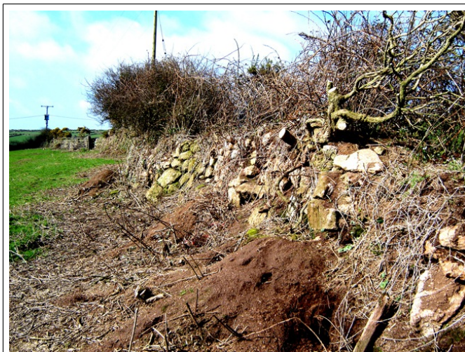
Typical rabbit damage to a neglected Cornish hedge, with earth from the inside of the hedge structure mined out into the field.
